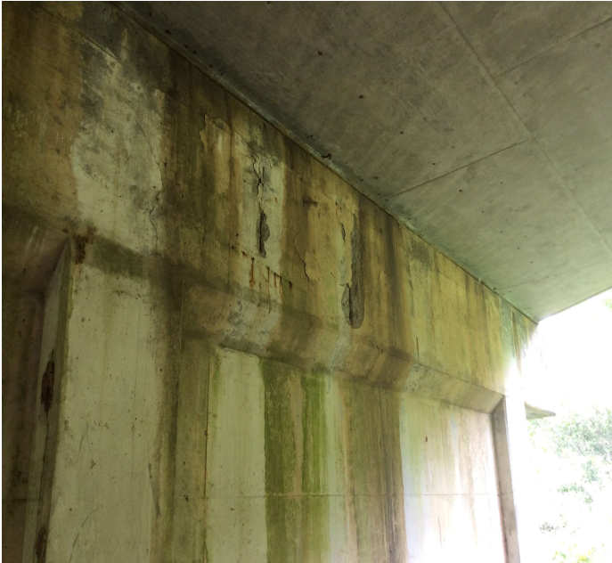
PHOTO 3 Description -Bent 5 has a large spall with exposed reinforcing steel on the ahead face of the cap near the centerline of the cap.
