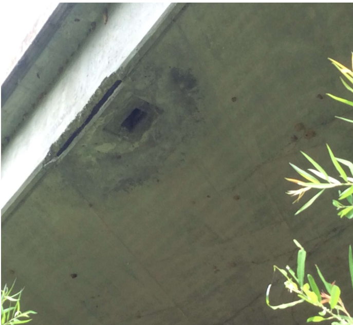
PHOTO 1 Description There is concrete spalling with exposed reinforcing steel around the deck drains visible from the undersurface.
