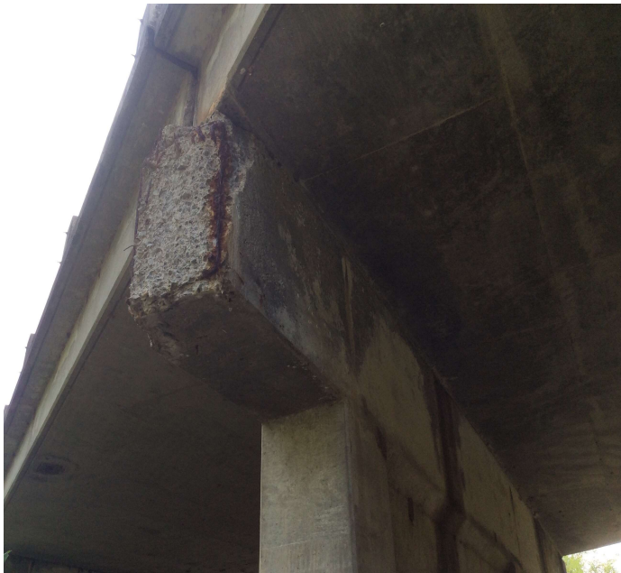
PHOTO 1 Description -Bent 4 has concrete deterioration with section loss and exposed reinforcing steel on the Lt end of the cap.
