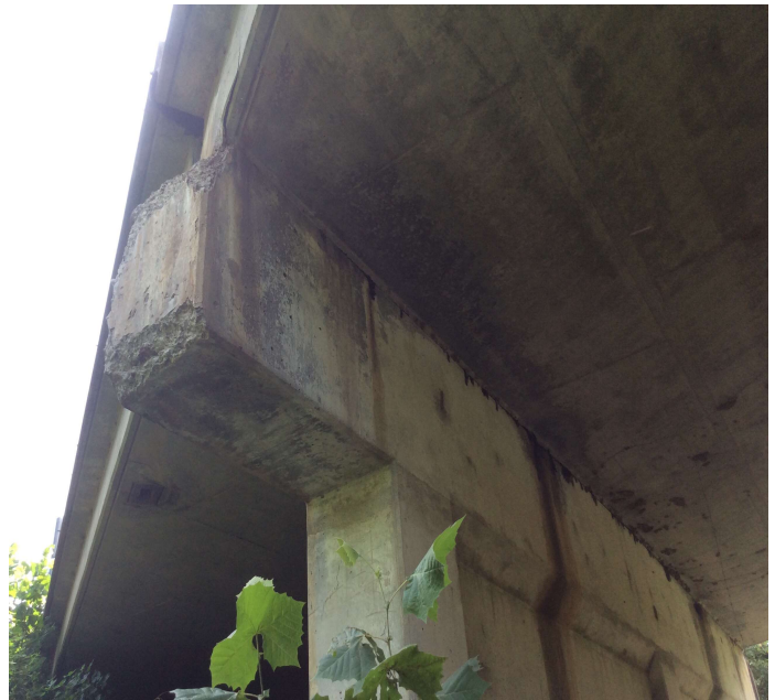
PHOTO 2 Description -Bent 5 Lt side has concrete deterioration with exposed reinforcing steel.
