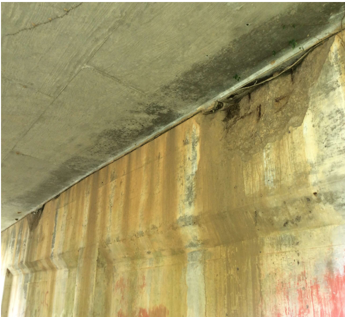
PHOTO 4 Description -Bent 2 has a 3' wide spalled area on the Rt side of the cap at the keyway. -Bent 2 has has a 3' spalled area on the Lt side of the cap with exposed reinforcing steel.
