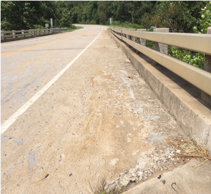
PHOTO 1 Description Deck The gutters have light / medium scale.
